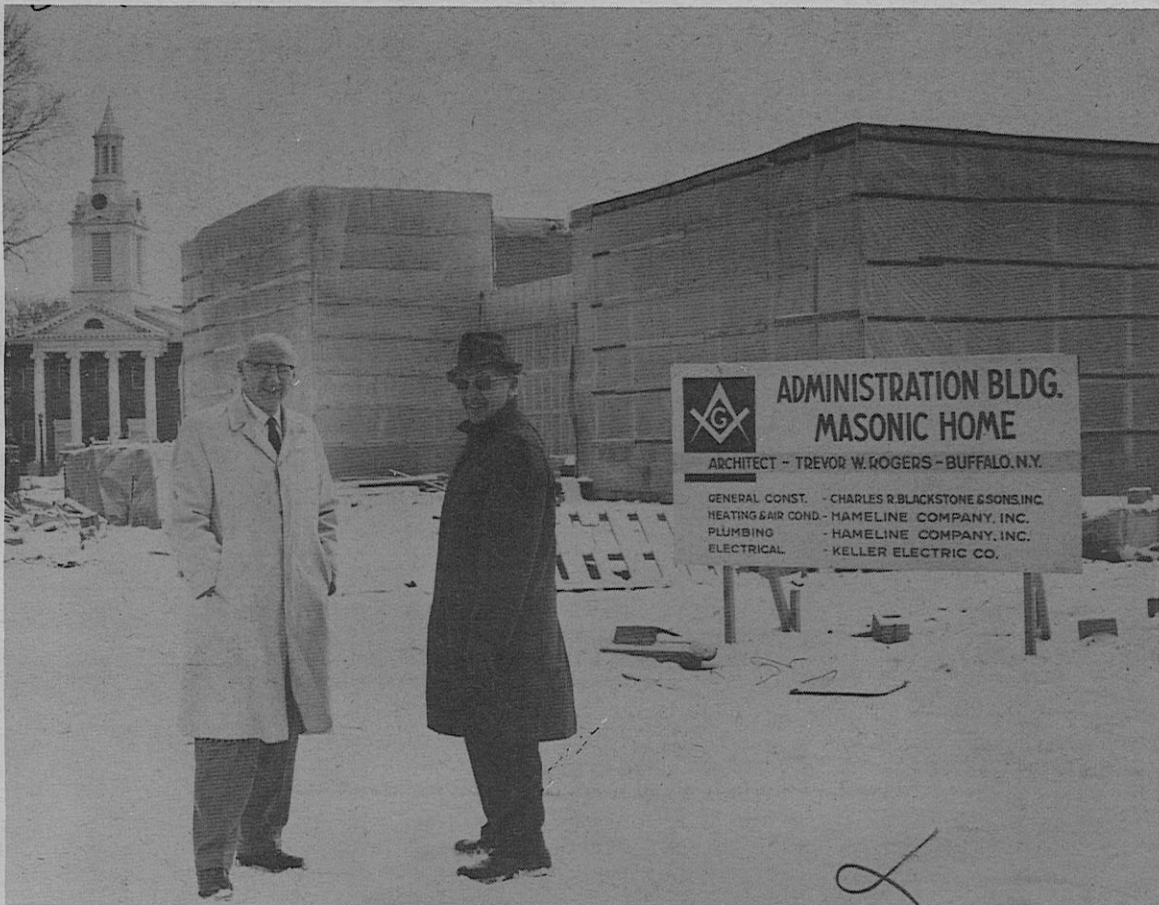
DR. WILLIAM T. CLARK , shows a visitor the new Masonic Home Administration Building scheduled for completion by early summer. The ultra modern single story structure, of steel marble brick and glass, will house administrative offices, a Trustee's office, a Grand Masters' office, the Superintendent's office, a parlor-conference area for receptions and meetings, and a 600 seat auditorium. Dedication is set for Saturday, June 18.
